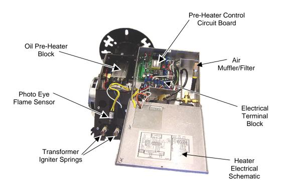
Figure 2 - Oil Burner (Back View Opened)
